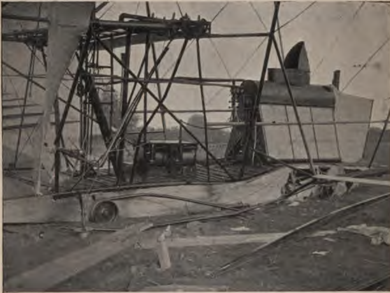
Fig. 81.—Shows the broken planks and the wreck that they caused. It will be observed that the wheels sank directly into the ground without leaving any track.
